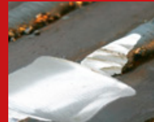
Remove of welding seams on steel
