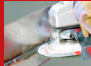
Processing of welding seams in angles
