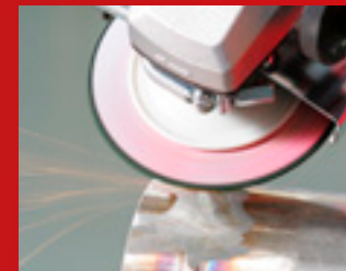
Remove and finishing of welding seams on stainless steel
